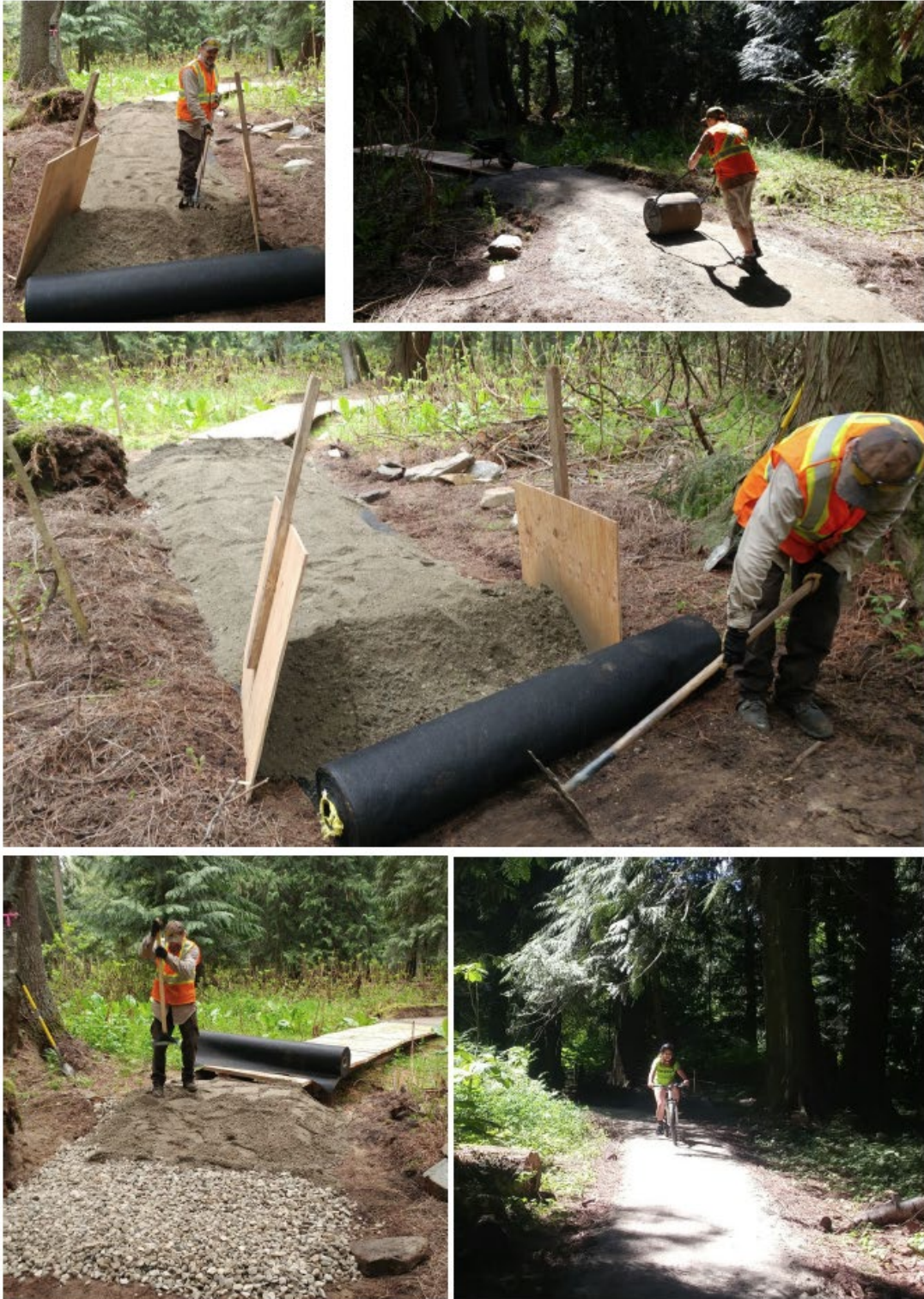
Plate 4.1-3. Example of the trail construction system proposed by the East Shore Trail and Bike Association.
